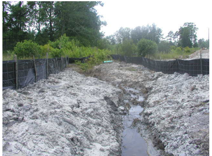
Facing Upstream from Culvert at end of Upper Reach
