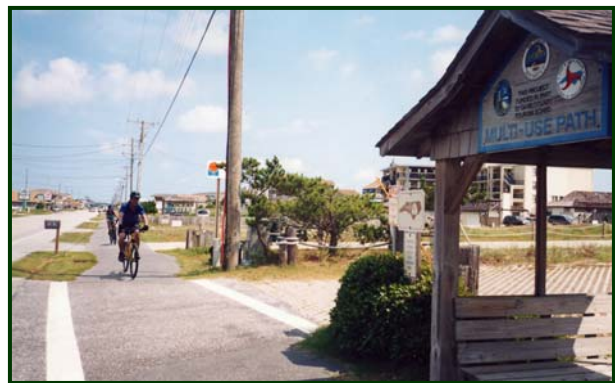
Nags Head Side Path – an off-road facility. Photo courtesy of NCDOT
